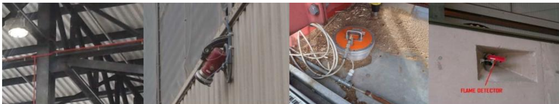
Left to right: Aspirating detector (red pipework) at a waste recovery site, visual type detector in external use overlooking a waste storage bunker, specialised gas detector at a wood chip storage silo, flame detector set in a waste bunker wall
