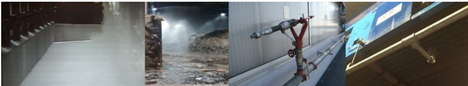
Left to right: Large foam system under test at a waste recovery plant, sprinklers in action at a recycling plant, manual-use water monitor at a waste site, under-gantry sprinkler head and pipework at a recycling plant
